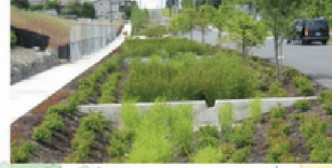
Stormwater Treatment Area
