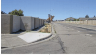
Banyan Place Intersection
