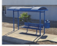
Bus Stop with Shelter
