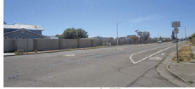
Wide Open Street Corridor
